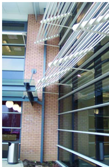
Marlborough House, Leatherhead. Solar C louvre installed onto Colt glazed pyramid with integrated Colt Firelight ventilators.
