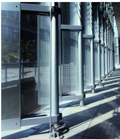
UTZ Offices, Berlin, Germany. Bespoke vertical solar shading fins that can be manually altered to control internal daylight levels.
