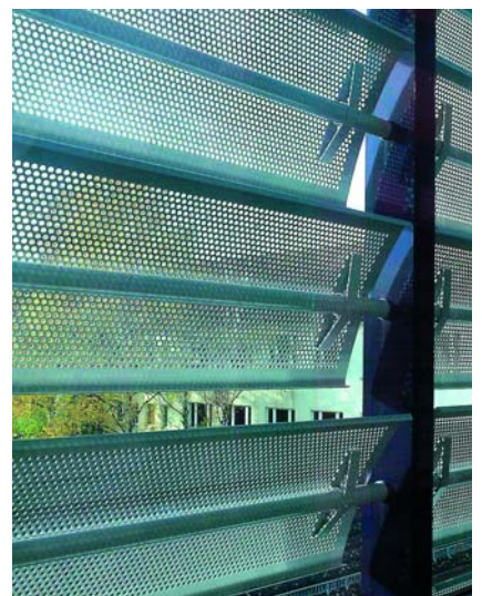
SD Worx, Germany. Controllable perforated Shadometal.
