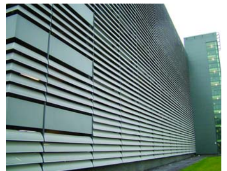
Addenbrookes Hospital, Cambridge. Perforated cladding and perforated Solarfin for screening and ventilation.
